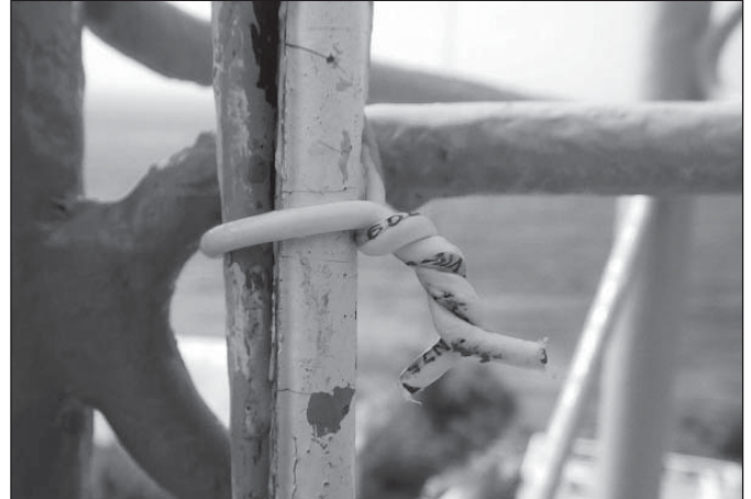
Figure 12 — Proper attachment of cables to towers in salty environments using #12 solid copper wire.
